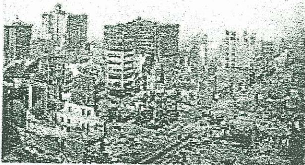
1906 San Francisco Earthquake
